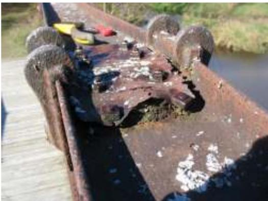
a badly corroded splice plate. The steel had rusted to the point where it was flaking apart and expanded to several times its original thickness. That discovery triggered an inspection of other splice plates, revealing nearly all were badly corroded.
