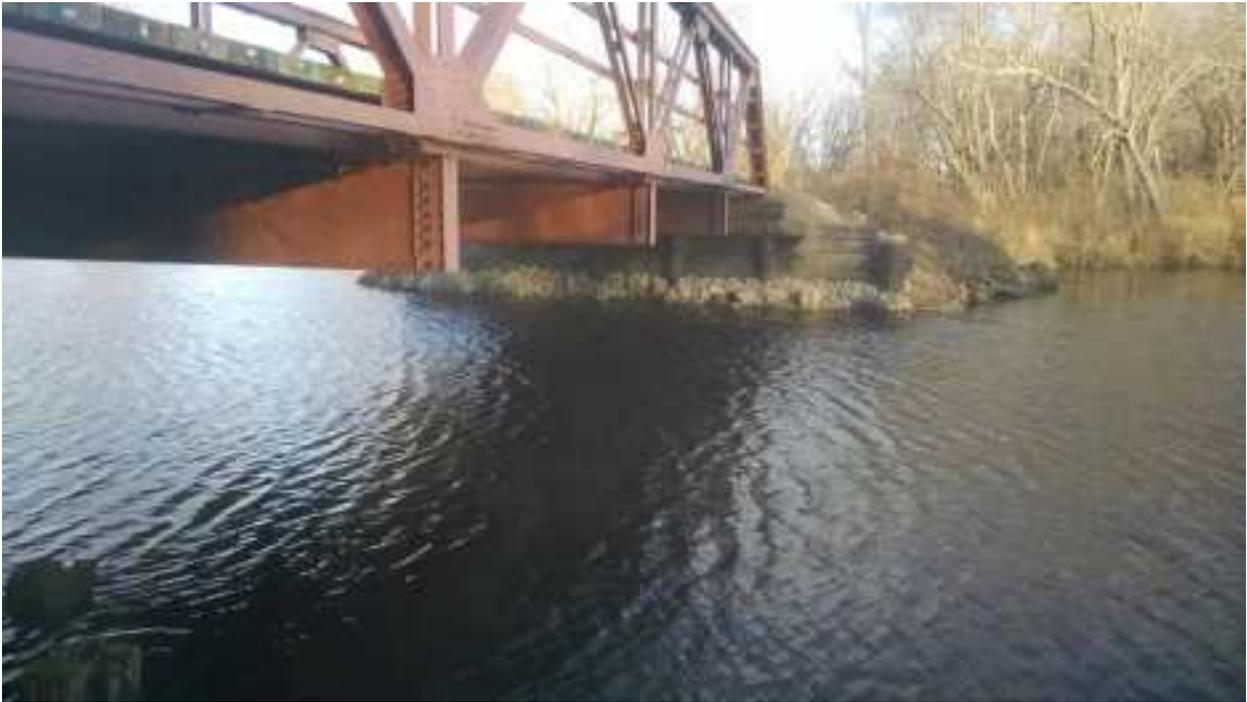
They added about 30 to 40 yards of river rock to Bridge 5's abutment. It is estimated to be about 35 feet deep in the middle of the river channel. Yikes!
